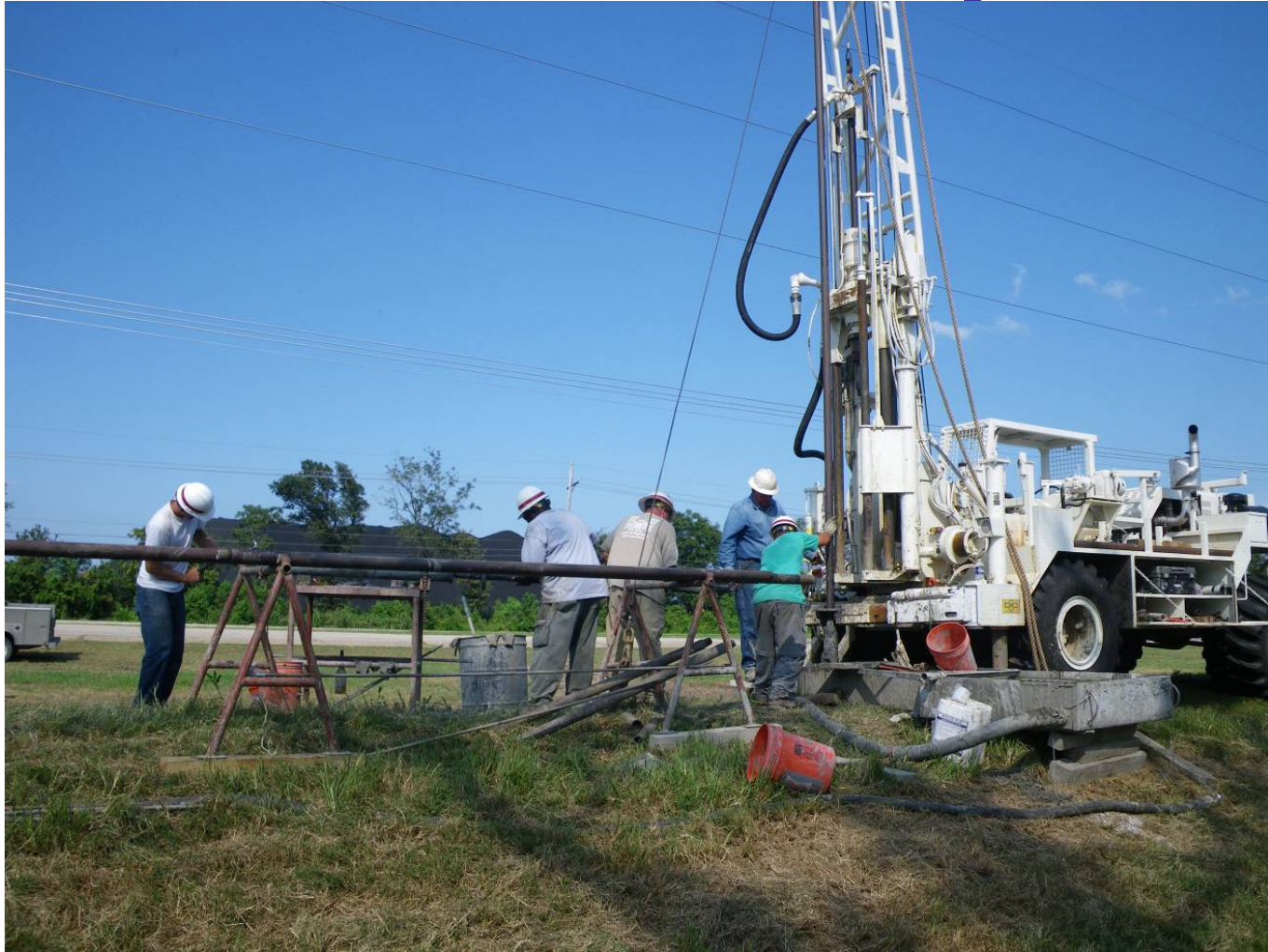
Soil Boring Rig
